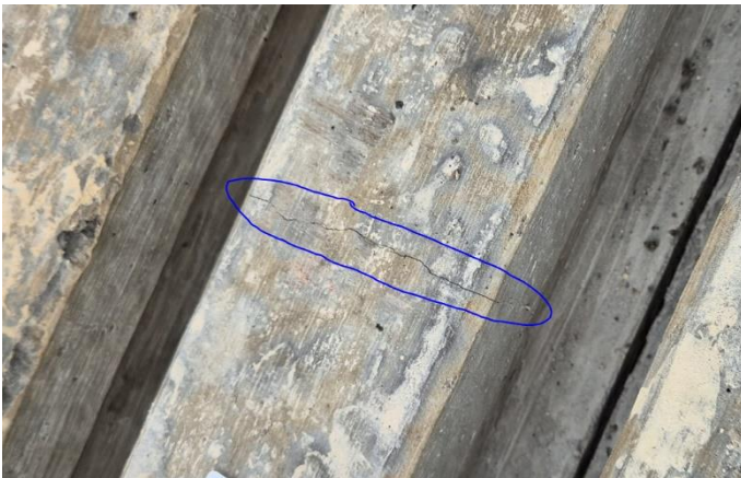
Figure 1 – micro crack present on top surface
