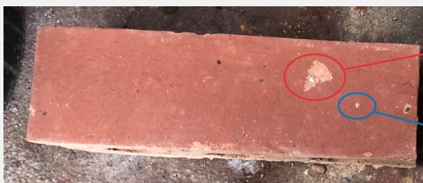
Figure 1 – Lime disruptions to the face of the brick.
