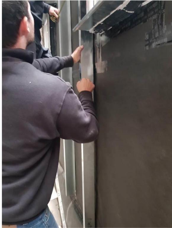
**Plate 8** – Installation of Zed Rails
