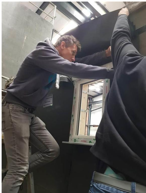
**Plate 5** – View of Installation of Breather Membrane
