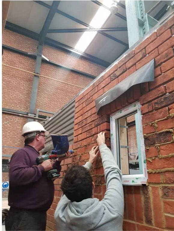
**Plate 12** – Application of Pointing Mortar
