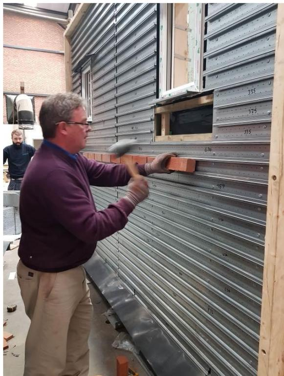
**Plate 11** – Installation of Brick Slips
