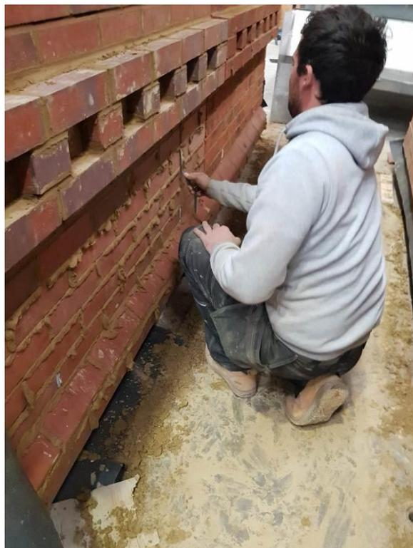
**Plate 13** – Finishing of Mortar Joint
