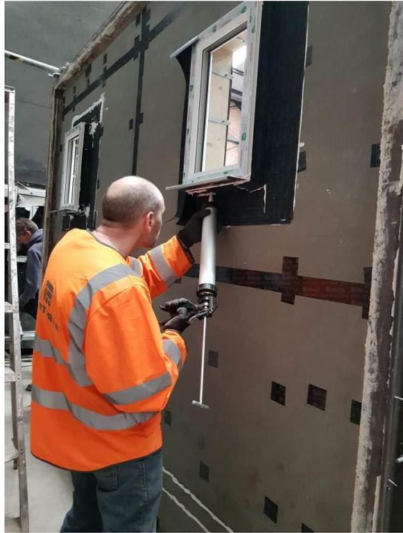
**Plate 4** – View of the 'DPC Installed to Window Perimeter and Cement Particle Board
