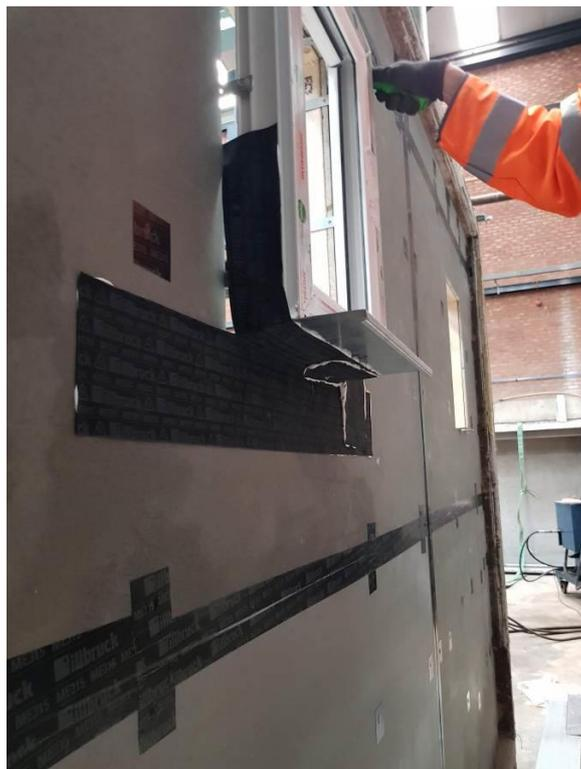
**Plate 3** – View of the 'DPC Installed to Window Perimeter
