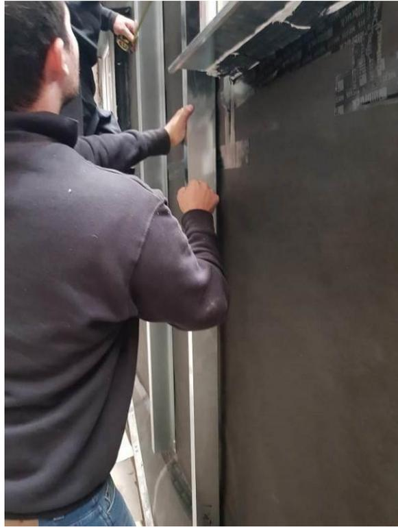
**Plate 8** – Installation of Zed Rails
