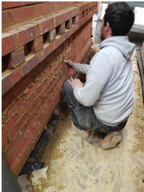
**Plate 13** – Finishing of Mortar Joint
