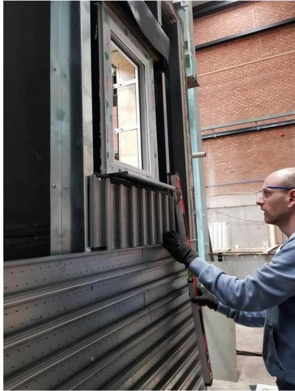
**Plate 10** – Installation of Brick Rail
