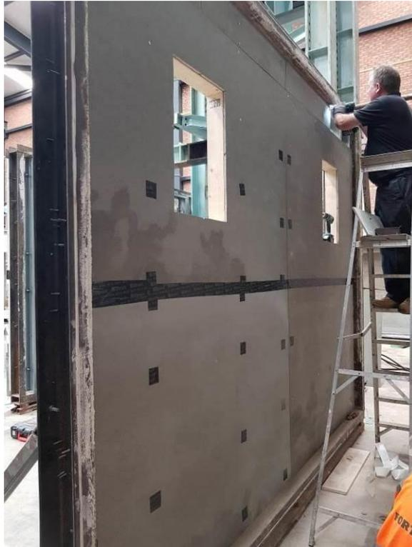
**Plate 2** – View of Joint Taping Cement Particle Board
