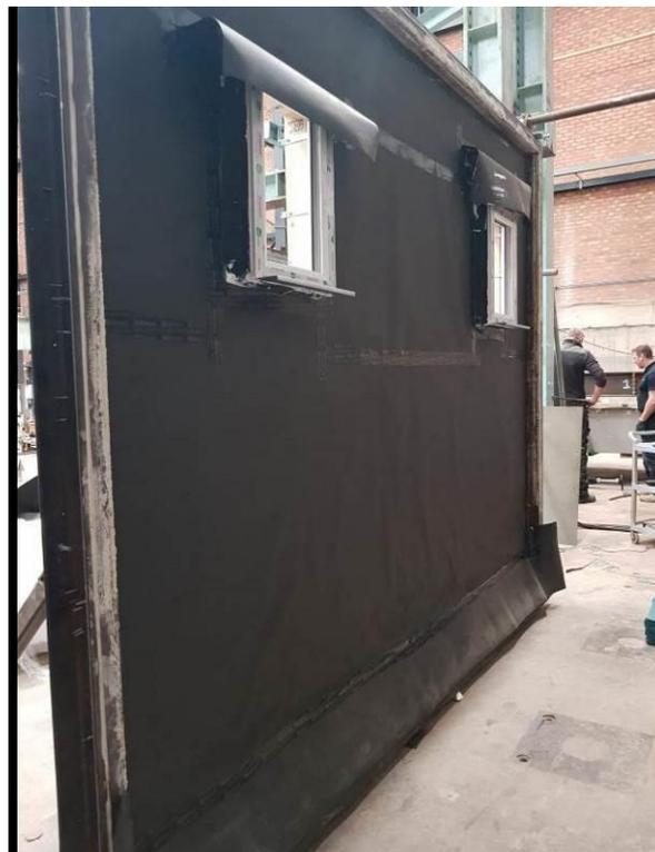
**Plate 7** – Wall after Installation of Breather Membrane
