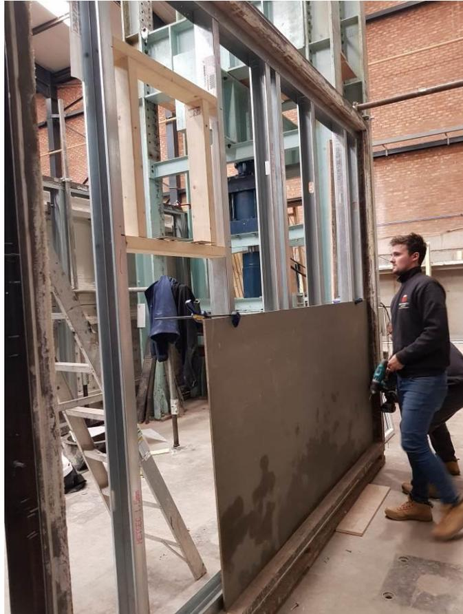
**Plate 1** – Mechanically Fixing of the Cement Particle Board onto the Galvanised Metal Frame Previously Installed
