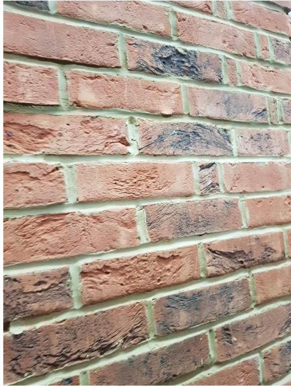
**Plate 14 – Finished of Joints**
