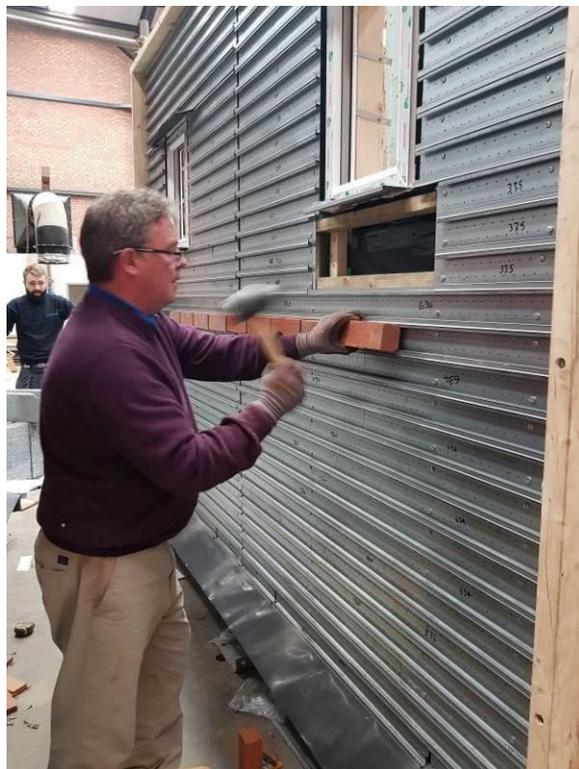
**Plate 11** – Installation of Brick Slips
