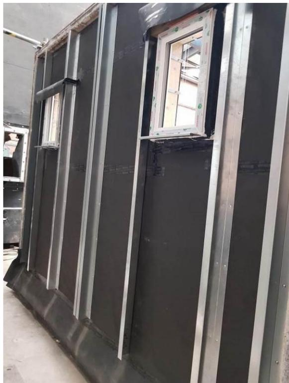
**Plate 9** – Wall on Completion of Zed Rail Install
