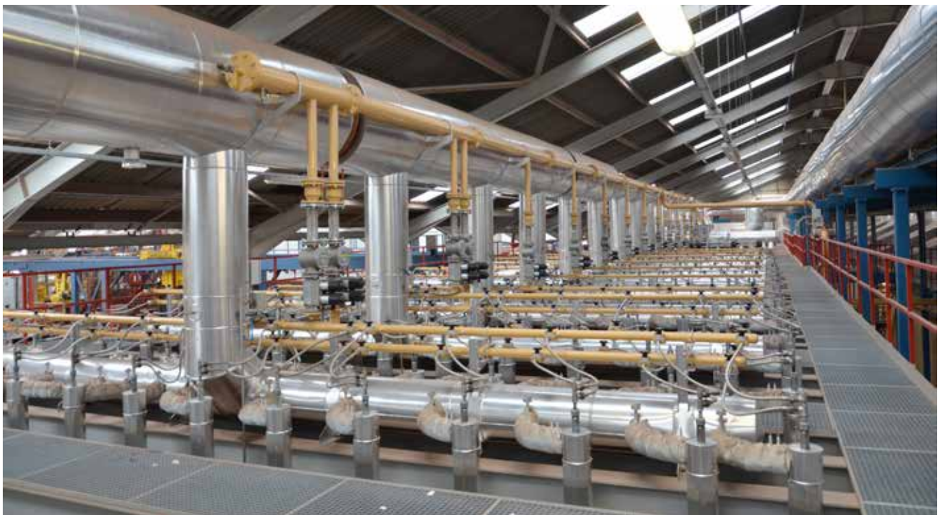
Top of Tunnel Kiln
