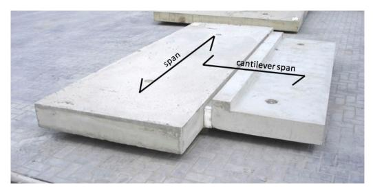
Figure 3 – Plan view of balcony slab cast with integral backspan slab.
