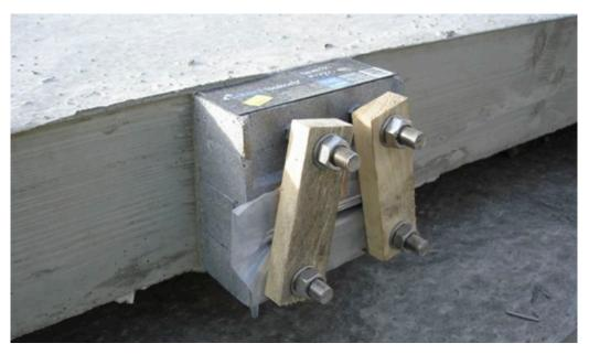
Figure 2 – Close up of cast in thermal breaks.
