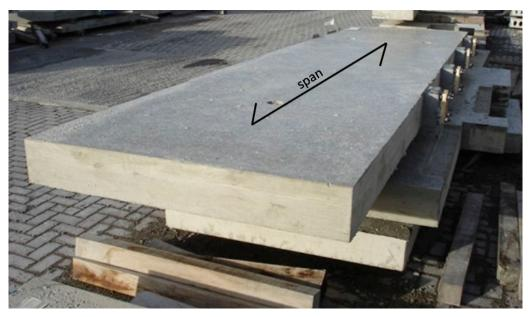
Figure 1 - RC landing slab with 4No. cast in thermal breaks.
