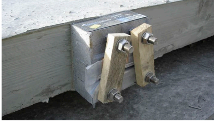
Figure 8 – Close up of cast in thermal breaks.
